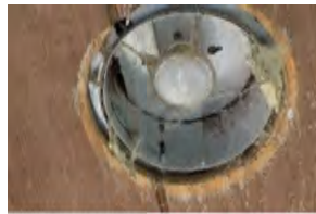
513 Allen's Creek Footbridge
