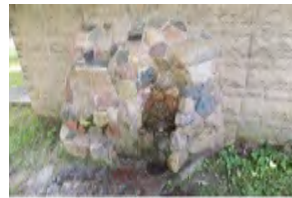
6 Leonard Park Bathroom Buil
