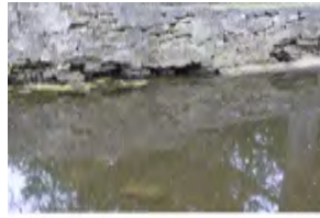
Creek Rip-Rap Horseshoe La
