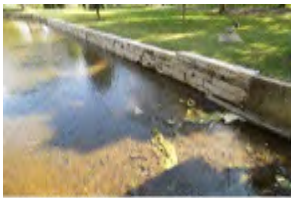
601 Allen's Creek Rip-Rap
