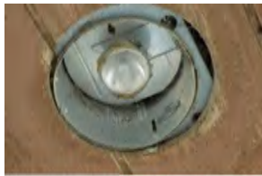
512 Allen's Creek Footbridge
