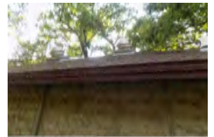
7 Leonard Park Bathroom Buil
