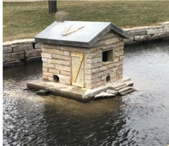
Figure 2.3: Restored Duck House in 2020
