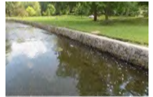
610 Allen's Creek Rip-Rap
