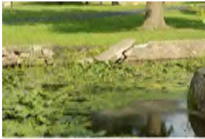
Allen's Creek Rip-Rap at East L
