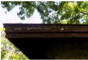
8 Leonard Park Bathroom Buil
