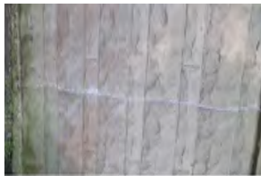
4 Leonard Park Bathroom Buil
