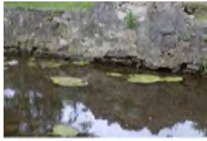
Creek Rip-Rap Horseshoe La
