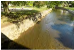
602 Allen's Creek Rip-Rap
