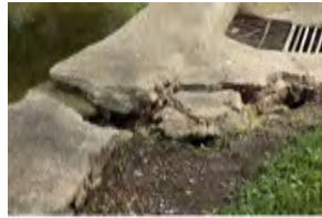
Allen's Creek Rip-Rap at East L
