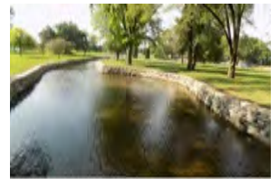
605 Allen's Creek Rip-Rap
