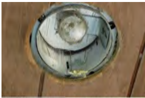
511 Allen's Creek Footbridge
