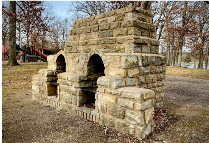
Figure 2.1 Leonard-Leota Park Rebuilt Fireplace in 2020
