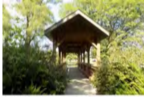
502 Allen's Creek Footbridge
