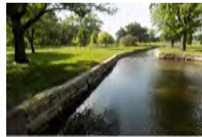
604 Allen's Creek Rip-Rap
