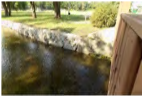
606 Allen's Creek Rip-Rap
