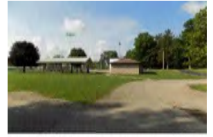
Diamond Bathroom Building & Office
