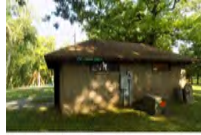
1 Leonard Park Bathroom Buil
