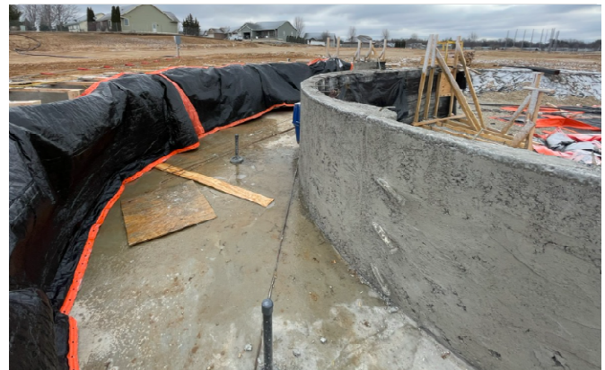
Forming continuing on river section walls
