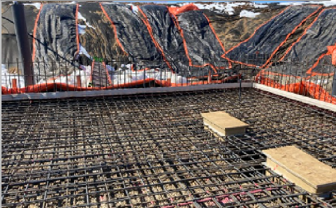
Rebar fully installed in lap pool floor
