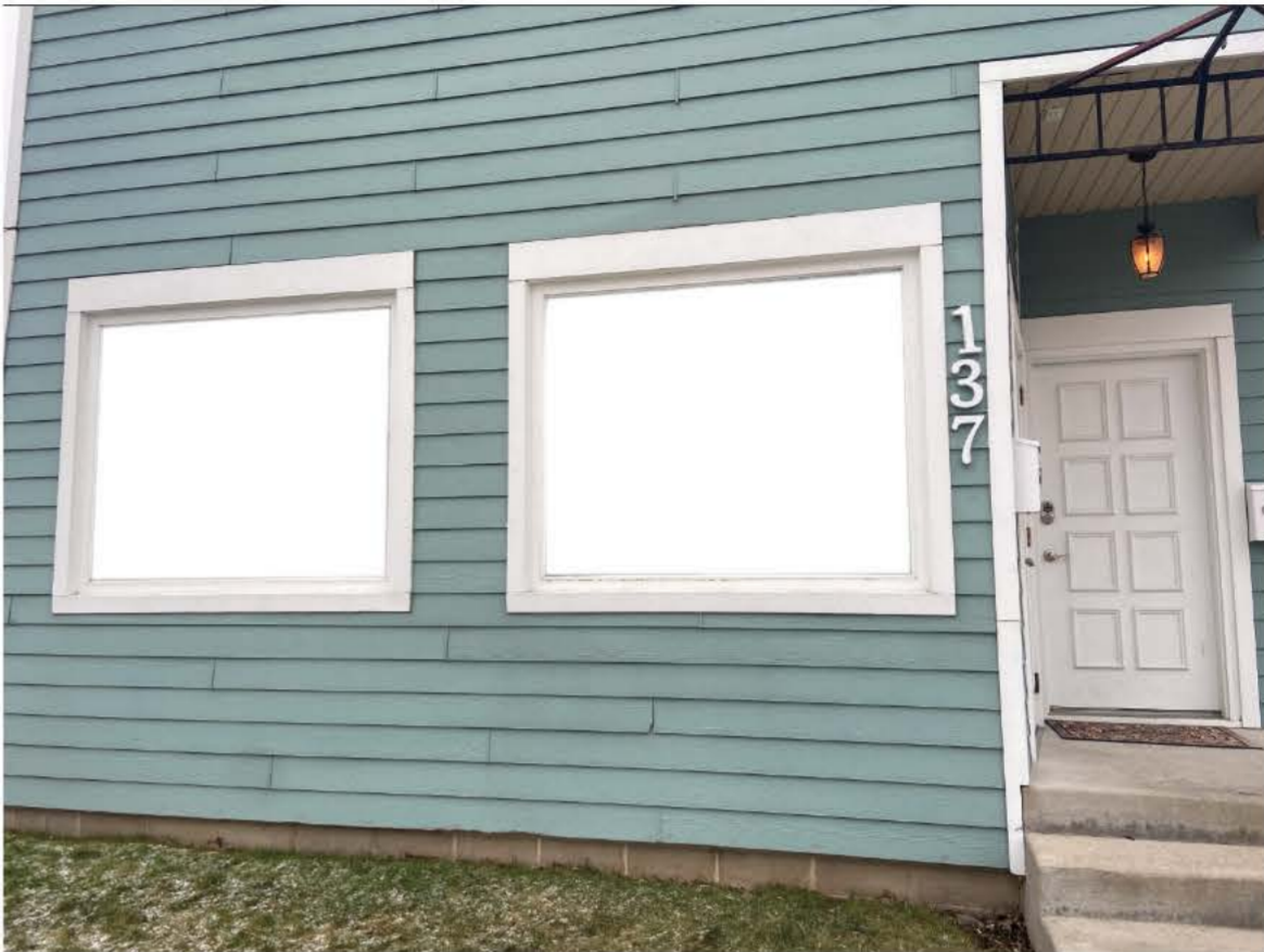
Front (north) view of building
