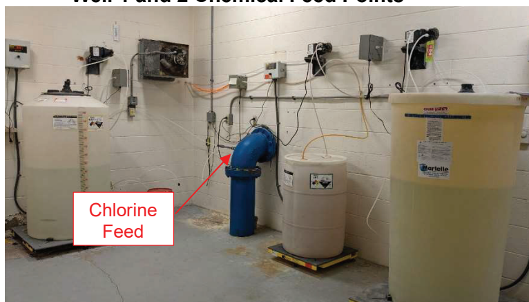
Well 1 and 2 Chemical Feed Points
