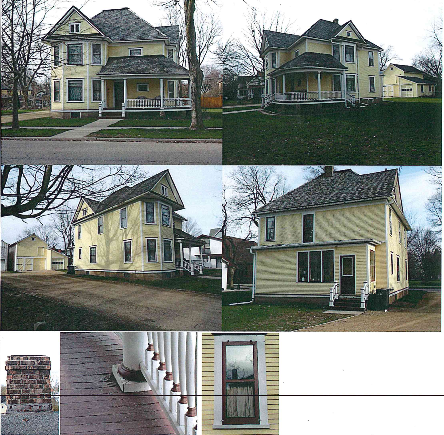
EXHIBIT: 1) Exterior Views, Current Chimney, Current Porch, Proposed Storm windows.
